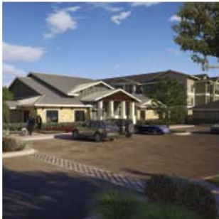
Oden Hughes has begun to build the 570-unit Landmark Southpark in Austin.
